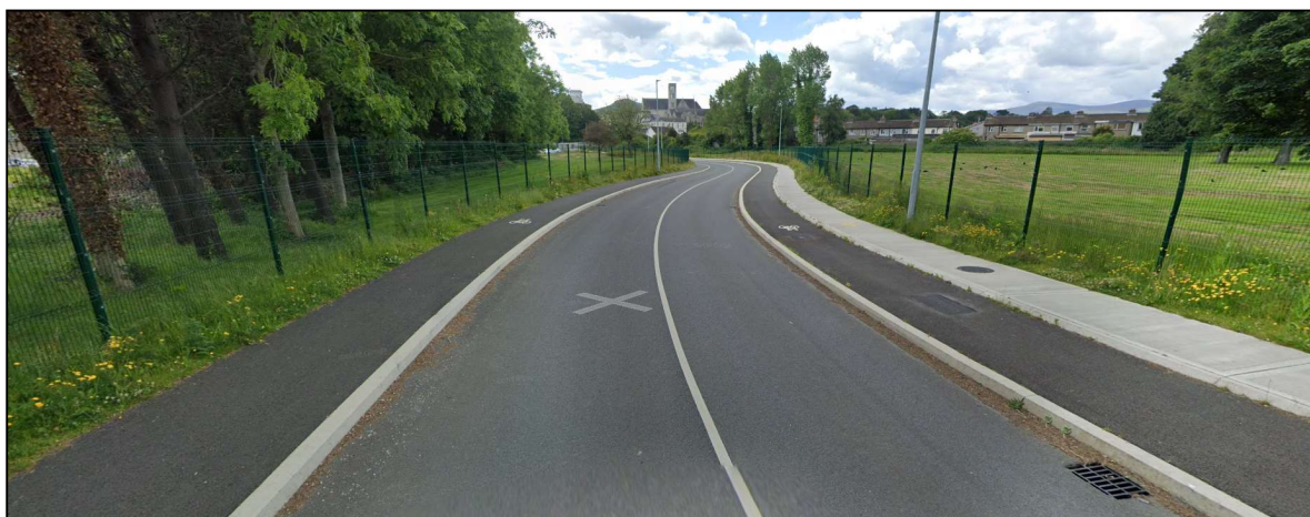
Figure 8-15 - Existing Southern Development Road
