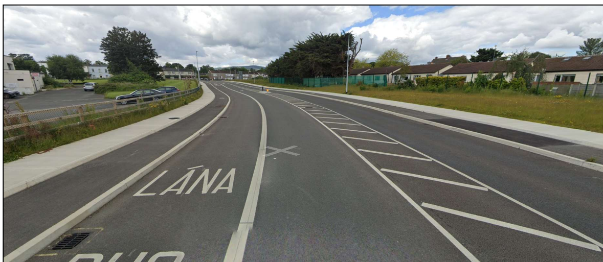
Figure 8-14 - Existing Northern Development Road
